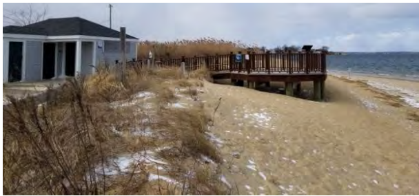
Millway Beach Bath House & Observation Deck
