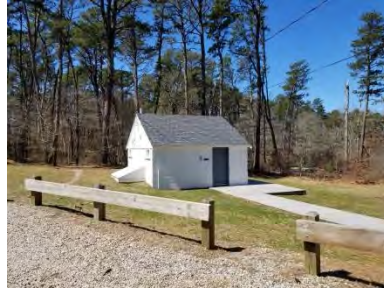
Hathaway's Bath House
