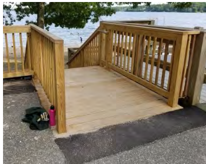
New Stairs & Handicap Ramp
