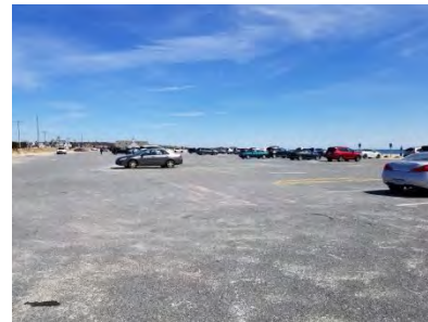
Craigville Parking Lot
