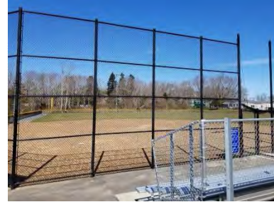
Lombard Field Fencing
